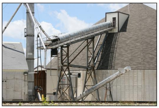
Structural design services provided for a steel frame supporting an industrial conveyor and catwalk used for unloading material from rail to a Dome Storage Building. The conveyor has a 45' cantilever span due to restrictions prohibiting any support within the Dome Storage Building. Structural analysis and design of the structural steel framing system and foundation support were provided. Required member sizes and connection details were provided to client.
