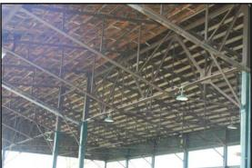
Project includes an inspection of the structural integrity of the Danville Stadium, built in 1946, including an in-depth inspection of the main timber structural framing members, a general evaluation of the secondary framing members and a complete inspection report detailing the type, extent and location of significant deterioration along with recommendations for repair.
